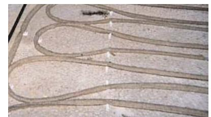
Another of the many advantages of limecrete is its user friendliness when it comes to underfloor heating. Once the limecrete has set, it is an easy task to clip in under floor heating pipes and to then install the screed and final floor finish.
